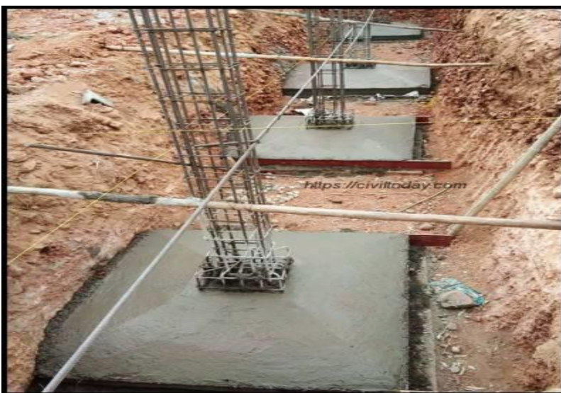
Figure 2 Isolated Shallow Foundation Image
