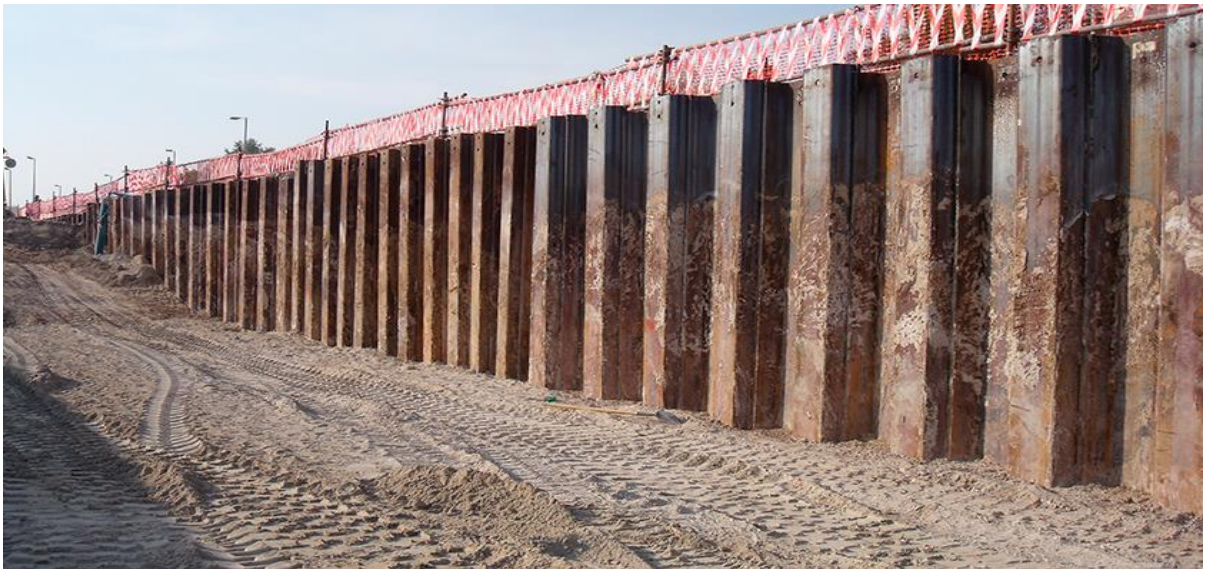
Figure 19 Sheet Pile Image
