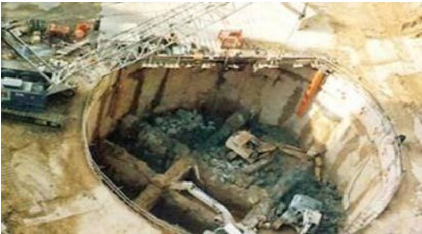
Figure 32 Excavated Caisson Image
