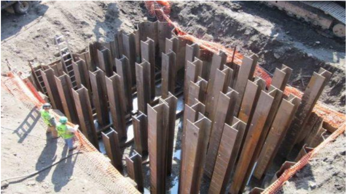
Figure 24 Steel Pile Image
