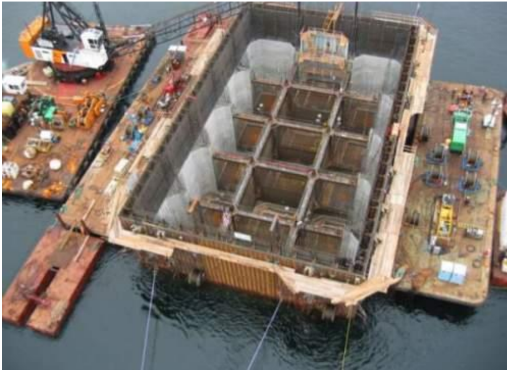
Figure 27 Caisson Foundation Image
