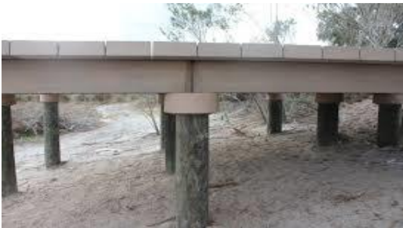
Figure 22 Timber Pile Image
