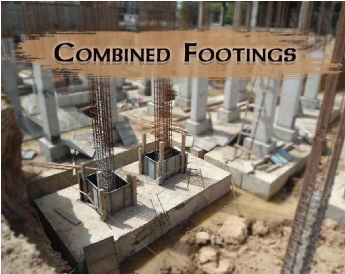
Figure 10 Combined Footing Image
