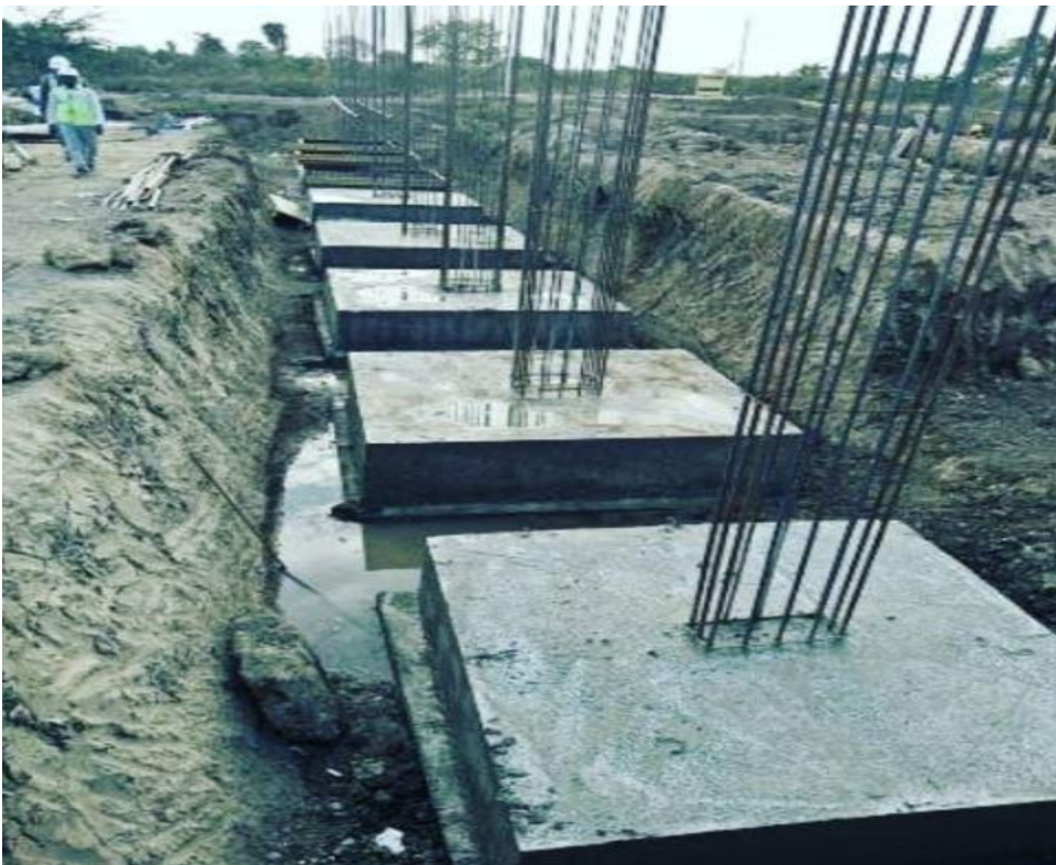
Figure 3 Single Pad Footing
